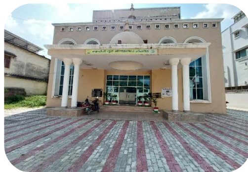
Shodhpeeth Road Construction & Setting up the idols of Nav Naths
