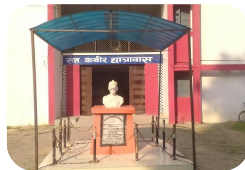
Major refurbishment of Sant Kabir Hostel (boys)
